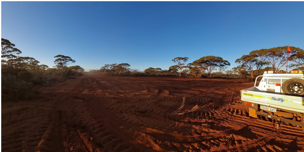
Limited preliminary site works by Versatile Plant Hire
