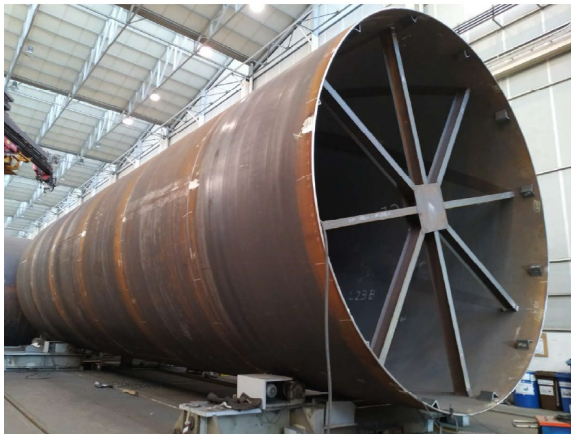
Rotary Kiln shell fabrication
