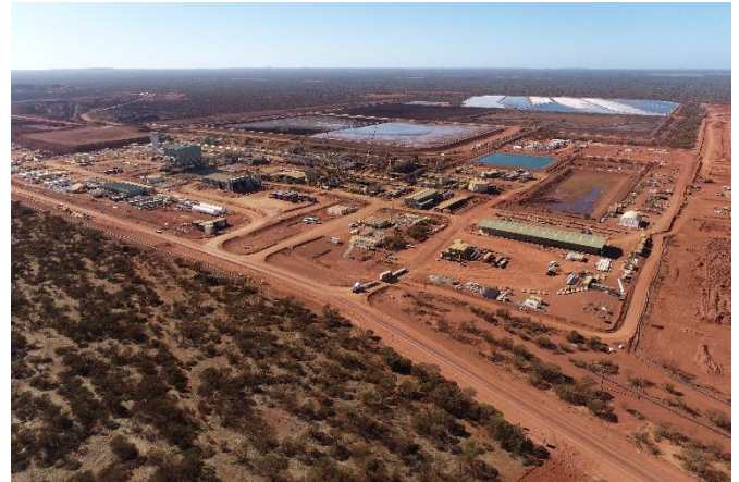
Drone photo of our Mt Weld expansion and operations
