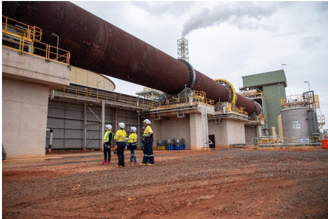
The kiln on site
